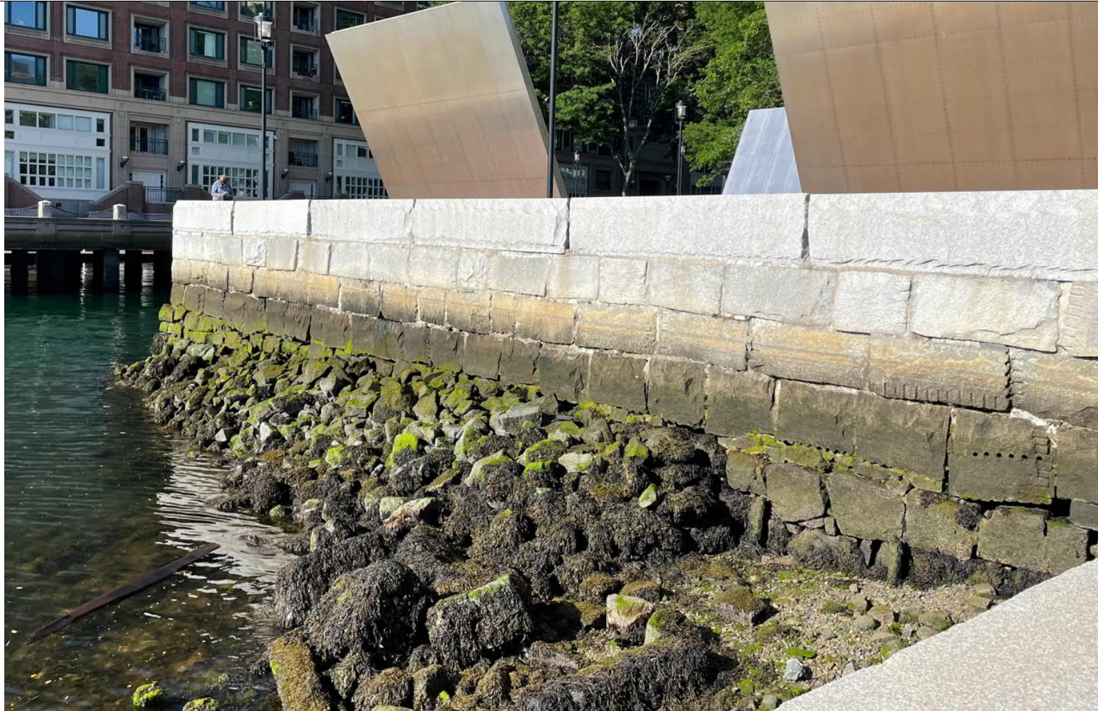
C – View of seawall (location 2)
