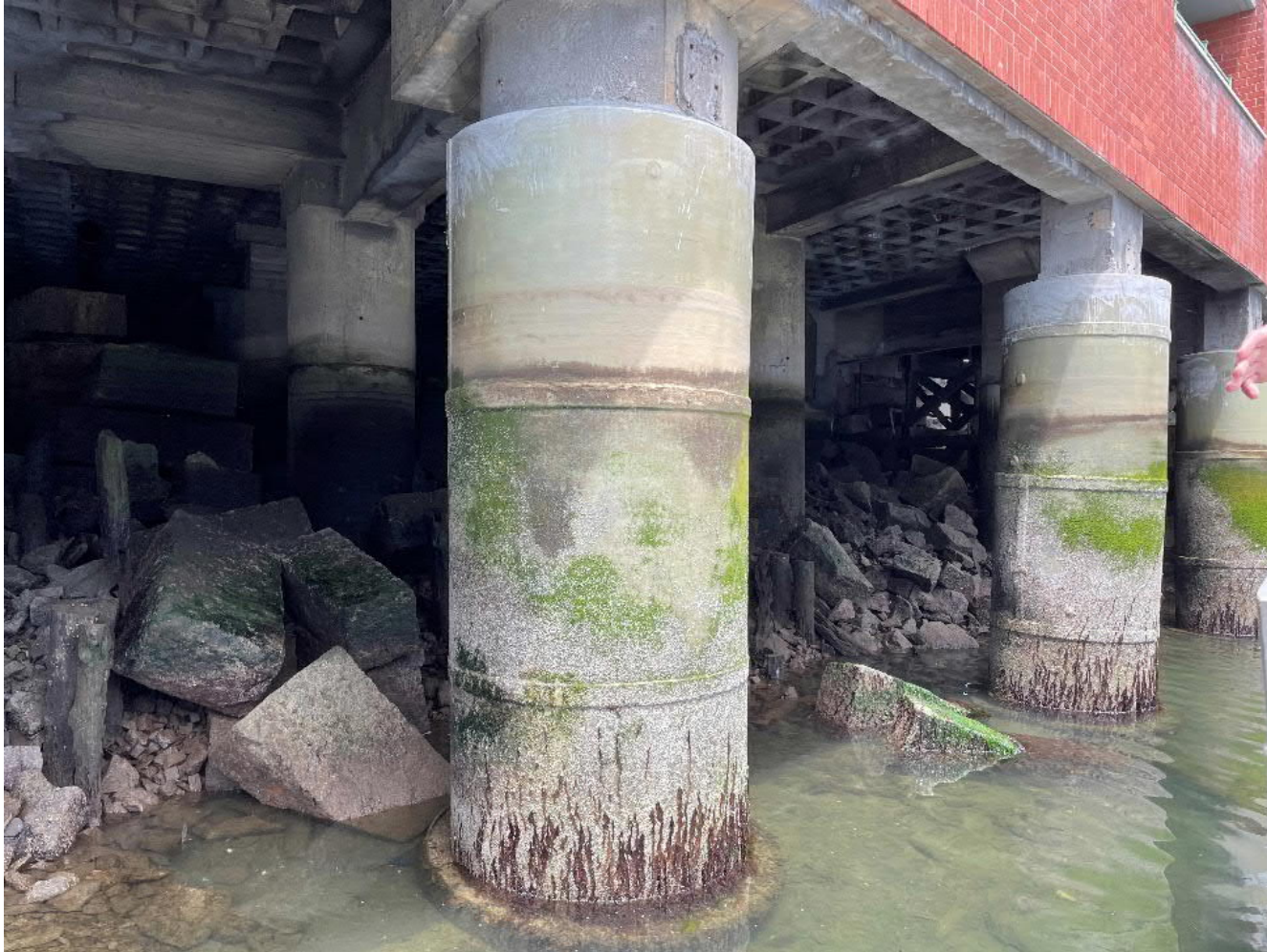
B – View of building supports
