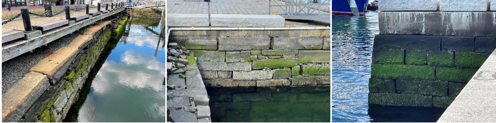
B – Typical South edge conditions – rebuilt granite seawall and existing granite seawall with concrete wall behind
