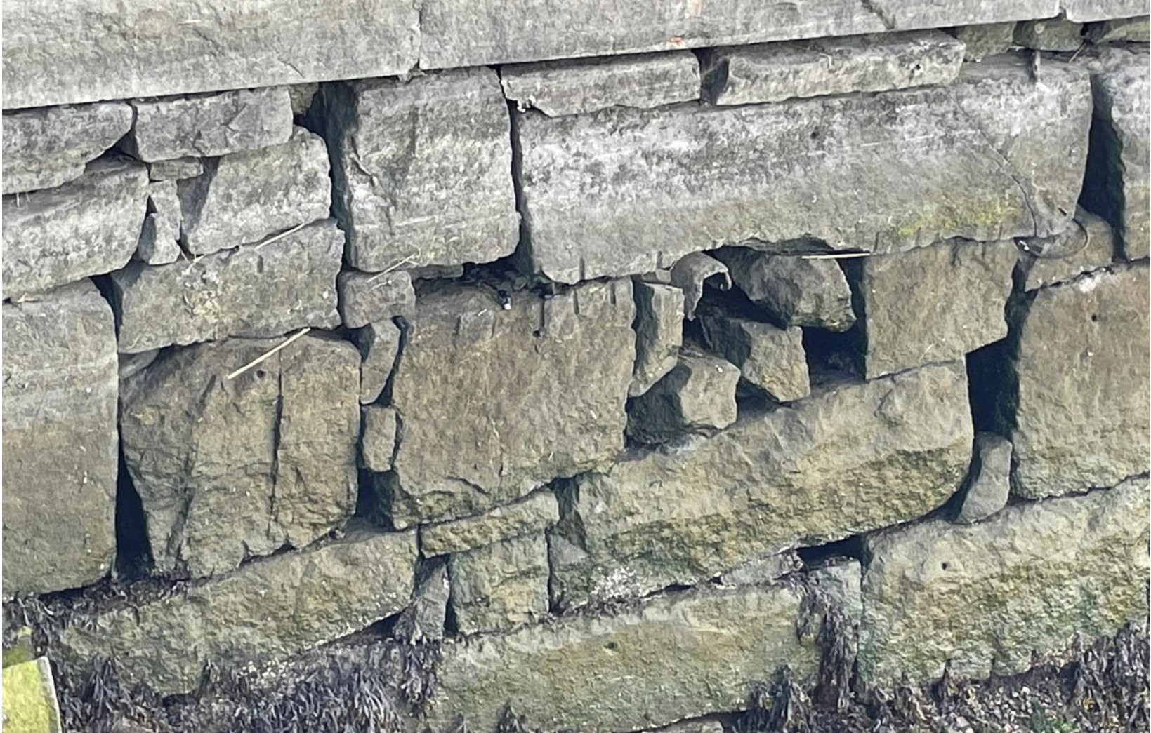
B – View of seawall, note some loss of blocks and opening of joints. Moderate portions have this level of damage.
