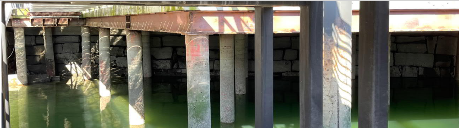
A – View of seawall
