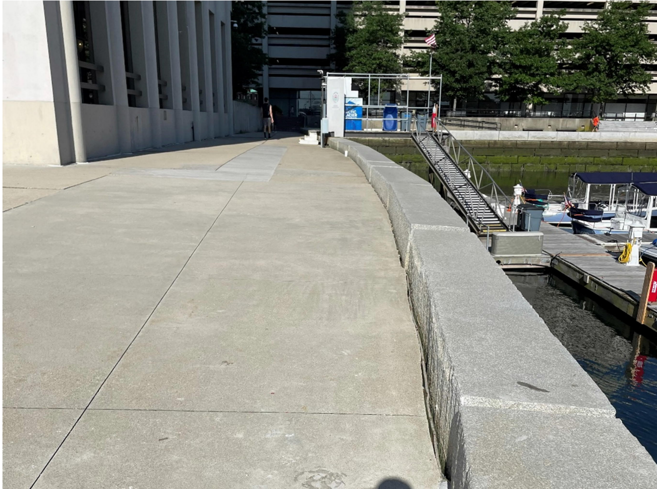
H – View of seawall (North edge)
