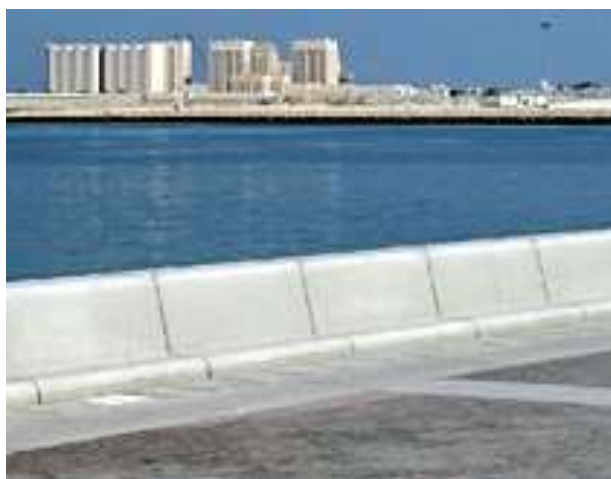
Figure 15. Example of parapet wall
