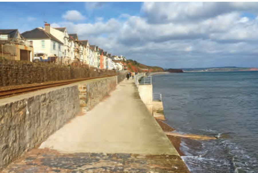
Seawalls are an example of a shore-based solution that can provide protection against storm surge as well as safe access to the ocean.
