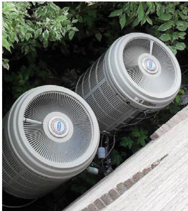
A residential air source heat pump. Photo credit: user Kristoferb/ Wikipedia
