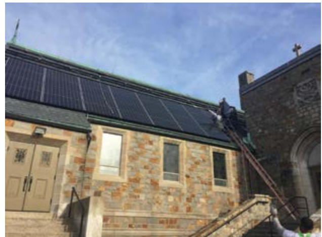
Solar Installation on Bethel AME Church in Jamaica Plain. Photo credit: Resonant Energy
