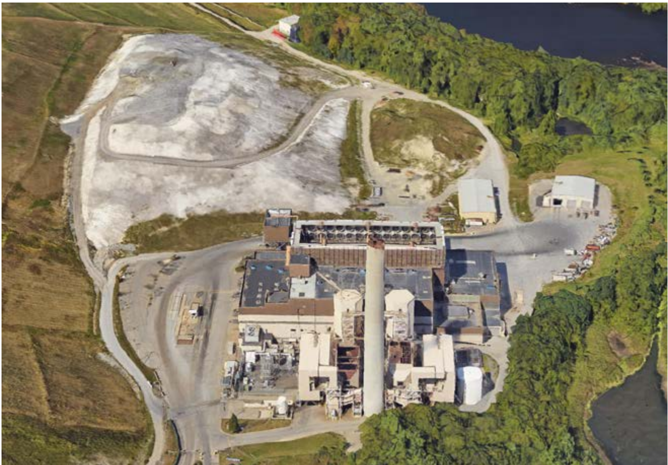
Covanta Haverhill waste-to-energy facility. Photo credit: Google Earth
